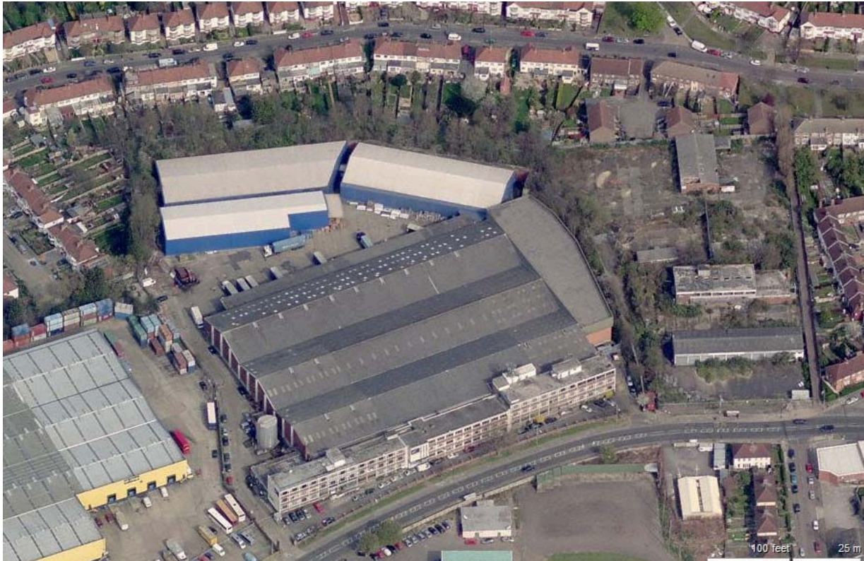
Figure 2: Aerial Photo of Previous Site Layout
